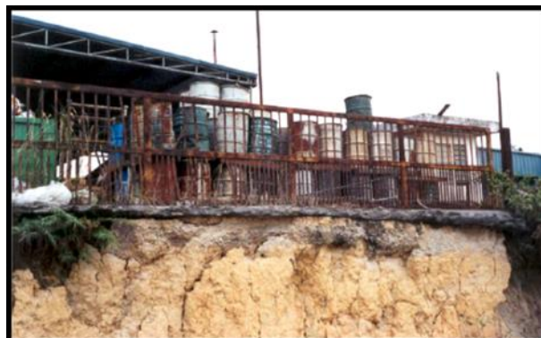
Plate 9.6.1: Example of Improper Storage of Scheduled Waste at the Edge of Slope
