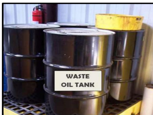
Plate 9.6.3: Storage Tanks for Waste Oil. The Capacity of the Containment Should be 110% of the Largest Containers Stored
