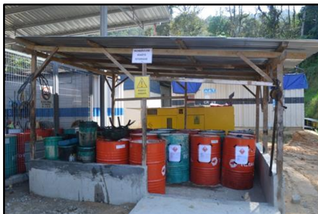
Plate 9.6.2: Example of Proper Storage of Scheduled Waste Labeling of Scheduled Wastes
